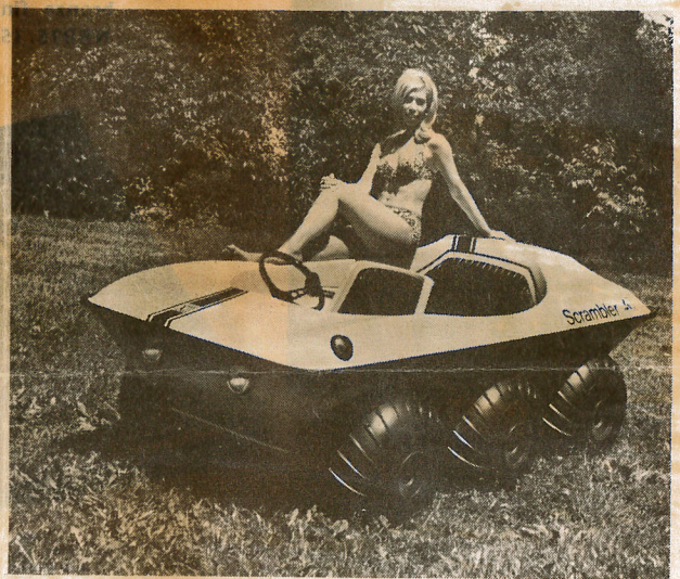
The Scrambler Marc XII. Runs in snow, sand, marshes, rough country and on the water.
